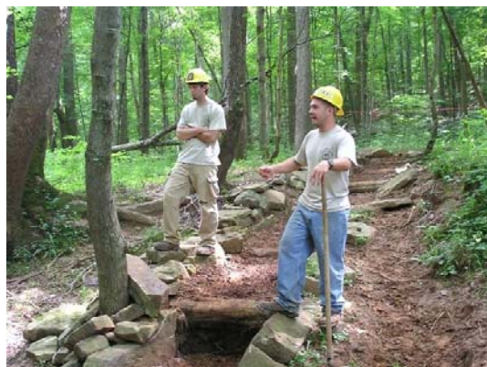
Wilderness Crew explain trail construction
